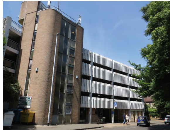
Photograph of existing car park
