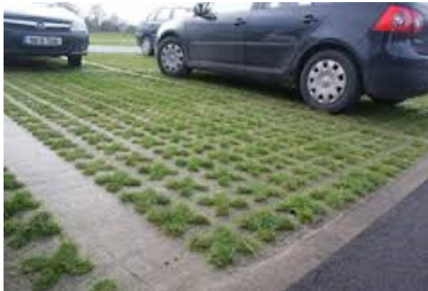
Fig 4. Grasscrete in use.
