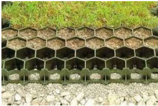
Fig 2. Close up of the grass reinforcement mesh
