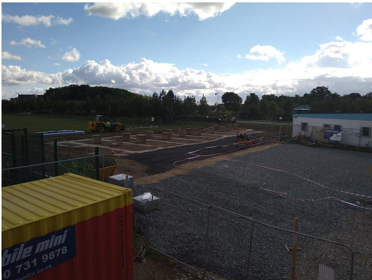
Progress as at 29th September 2021
