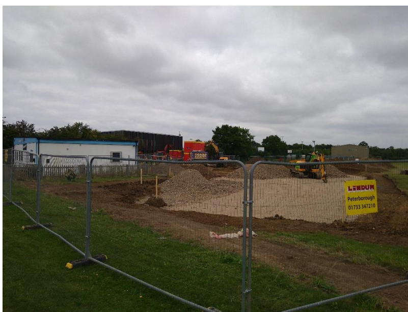
Site strip in preparation for excavating the Foundations 2/09/21
