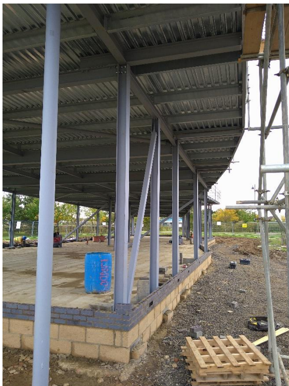
Progress as of 27 th October 2021
